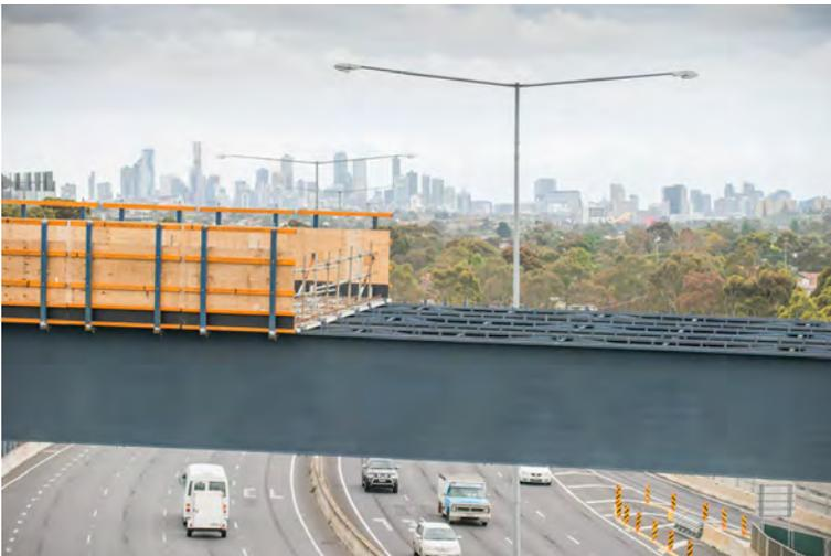
Later this month, the bridge deck will be complete when concrete is poured on top of the steel beams and panels crews installed throughout November and December.
