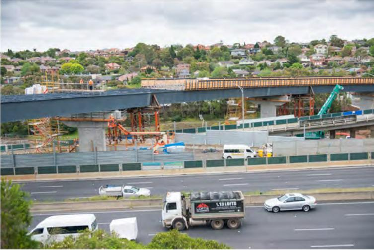
Under each of the bridge piers you can see in the above picture, an average of 10 piles were drilled in place to build the foundations for bridge.
