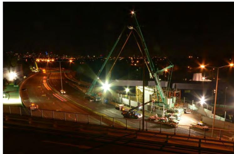
The three bridge beams installed across the freeway between 11 and 15 November are each two standard beams, joined on the ground to make a 'super beam', and lifted together using a 600 tonne, a 350 tonne and a 90 tonne cranes.
